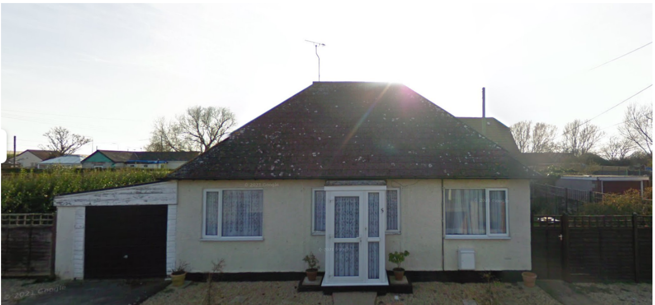
Figure 2: Photograph of the front elevation of the existing dwelling
